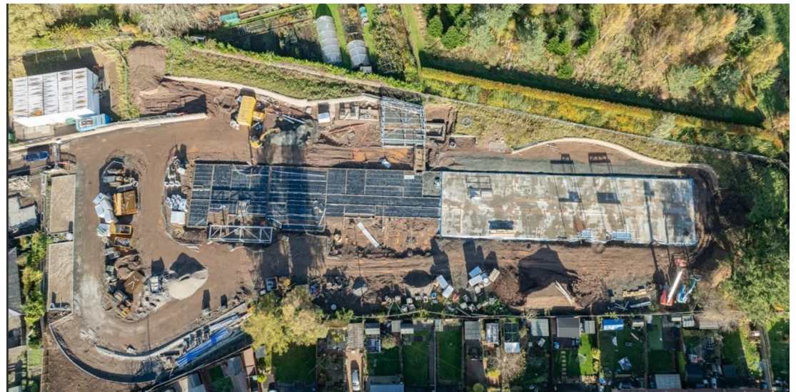
Work underway at Cupar Care Village
